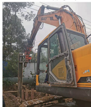
高压线下施工 Construction under high-voltage line
