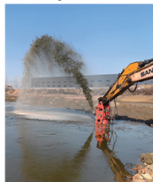
河道疏浚 River dredging
