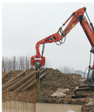
高铁承台钢板桩维护 Maintenance of steel sheet pile of high-speed railway cushion cap
