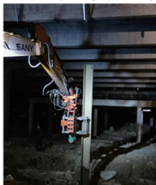
桥底施工 Construction under bridge
