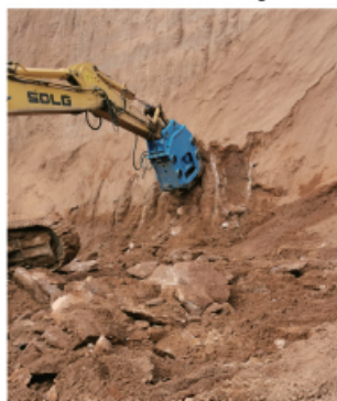
矿山施工 Mine construction
